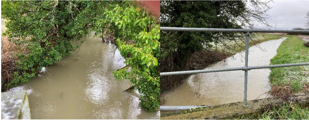
Washpit and Beck Brook, at time of highest water levels.
