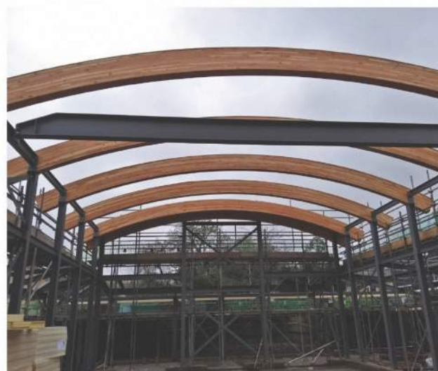
Glulam beams in place on the William Collyn Community Building.
